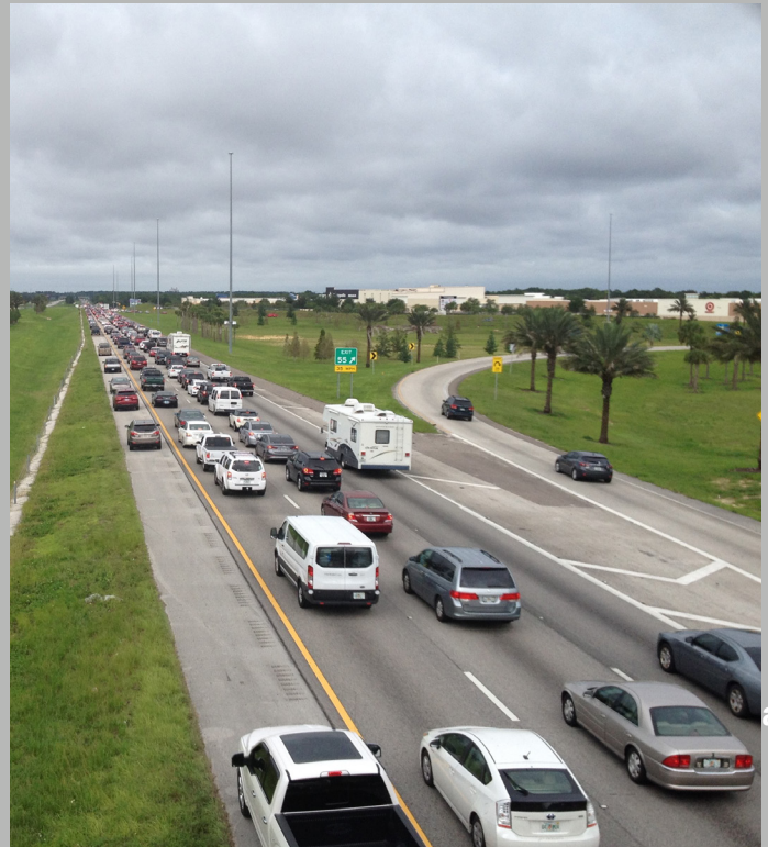
FIGURE 57: EXAMPLE OF HURRICANE EMERGENCY SHOULDER USE (ESU) GOING INTO EFFECT DURING FLORIDA'S HURRICANE IRMA
