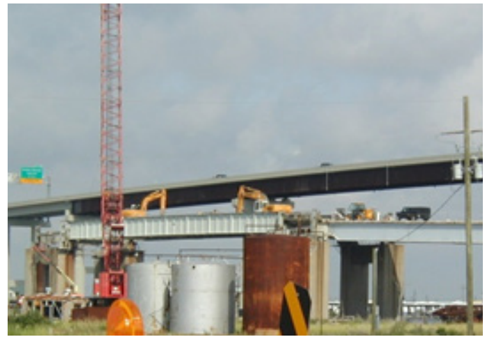
FIGURE 29: DEMOLITION OF THE LA-1 STRUCTURE IN LEEVILLE, LOUISIANA, AFTER CONSTRUCTION OF THE NEW BRIDGE. THE PROJECT INCLUDED THE DEMOLITION AND REMOVAL OF THE EXISTING LIFT-SPAN BRIDGE OVER BAYOU LAFOURCHE
