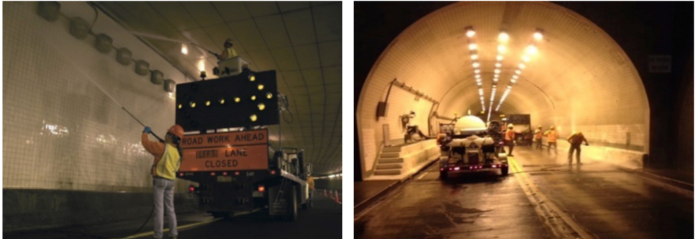
FIGURE 63: TUNNEL CLEANING CREWS IN ROSSLYN TUNNELS IN TEXAS
