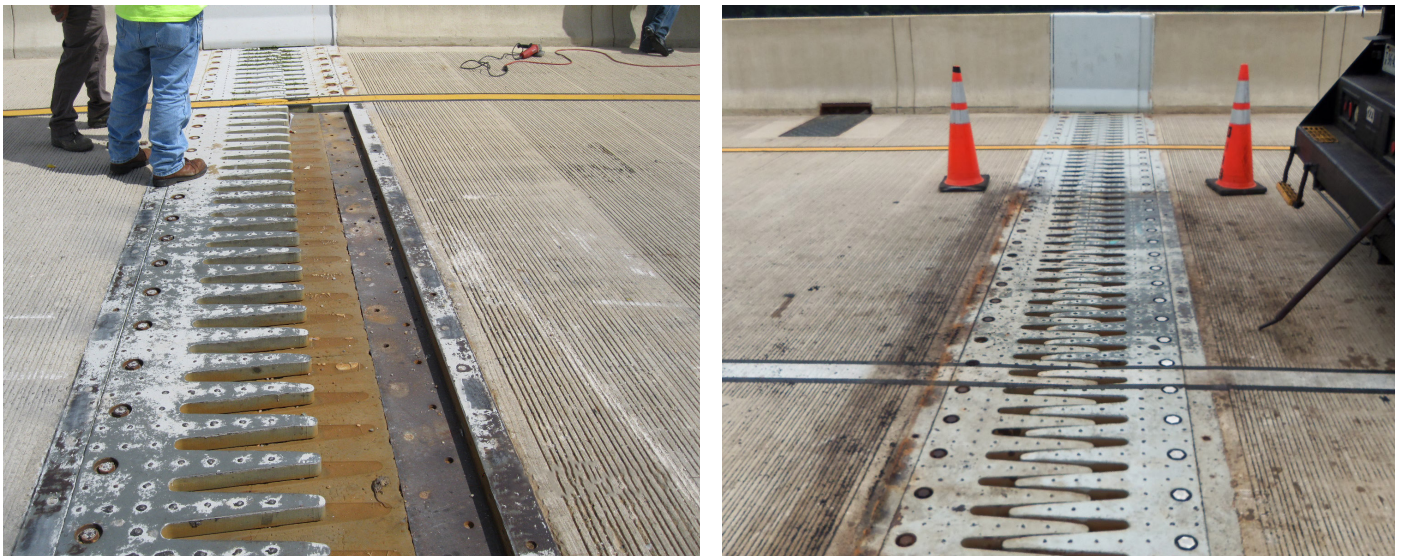
FIGURE 5 – EXAMPLES OF BEFORE AND AFTER FINGER JOINT REPAIR PICS-FL
