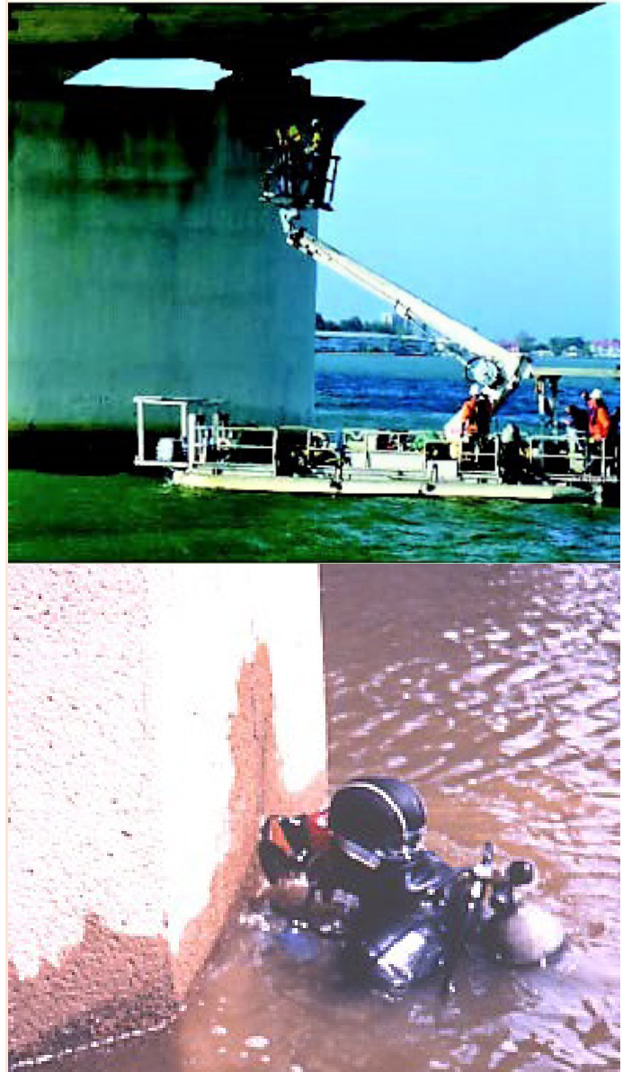
FIGURE 8: PIBC O&M TEAM MEMBER’S INSPECTION WORK
