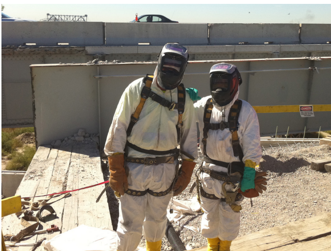
FIGURE 37: WORKERS PROTECTED AGAINST THE HAZARDS ASSOCIATED WITH LEAD-BASED PAINT DEMOLITION WORK ON THE CHRISTOPHER S. BOND BRIDGE PROJECT (LEFT) AND GALVESTON CAUSEWAY (RIGHT)
