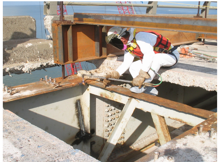
FIGURE 37: WORKERS PROTECTED AGAINST THE HAZARDS ASSOCIATED WITH LEAD-BASED PAINT DEMOLITION WORK ON THE CHRISTOPHER S. BOND BRIDGE PROJECT (LEFT) AND GALVESTON CAUSEWAY (RIGHT)
