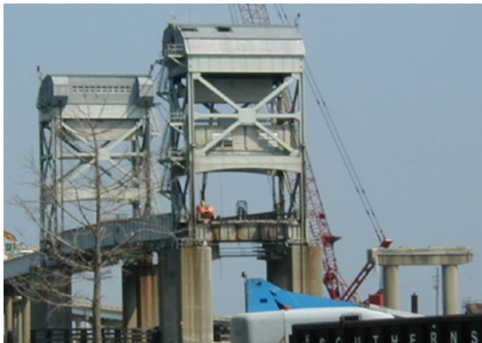
FIGURE 29: DEMOLITION OF THE LA-1 STRUCTURE IN LEEVILLE, LOUISIANA, AFTER CONSTRUCTION OF THE NEW BRIDGE. THE PROJECT INCLUDED THE DEMOLITION AND REMOVAL OF THE EXISTING LIFT-SPAN BRIDGE OVER BAYOU LAFOURCHE
