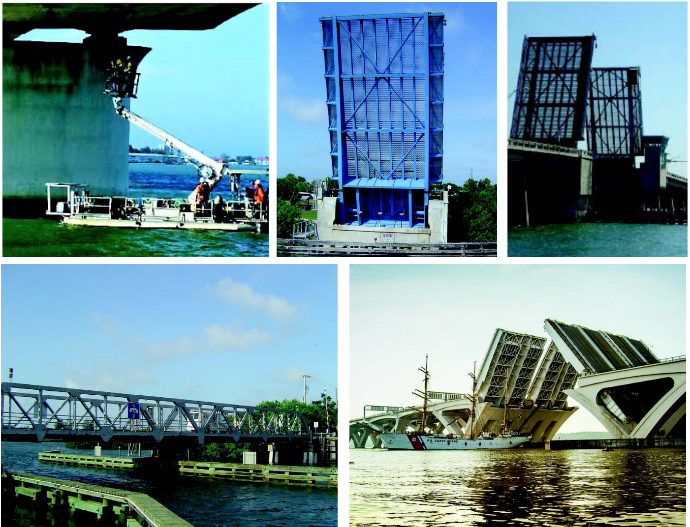
FIGURE 61: THE EXAMPLES OF OUR TEAM’S MOVABLE BRIDGE MAINTENANCE EXPERIENCE
